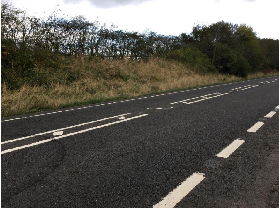
Plate 3-17 Stop 7 showing the cutting on the west side of the carriage way opposite the lay-by. Cutting is up to 2m high with a gradient estimated at 1V:2H.
